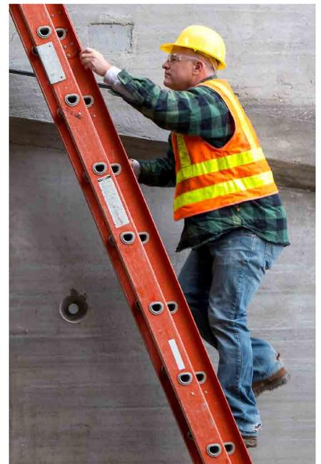
Three points of contact should be maintained when climbing or descending a ladder.
