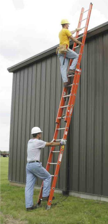
The workers have positioned the ladder to extend at least 3 feet above the point of support at the roofline. Until the ladder is tied-off at top and bottom (see “Securing the Ladder” on p. 8), the worker below must continue to secure it manually.
