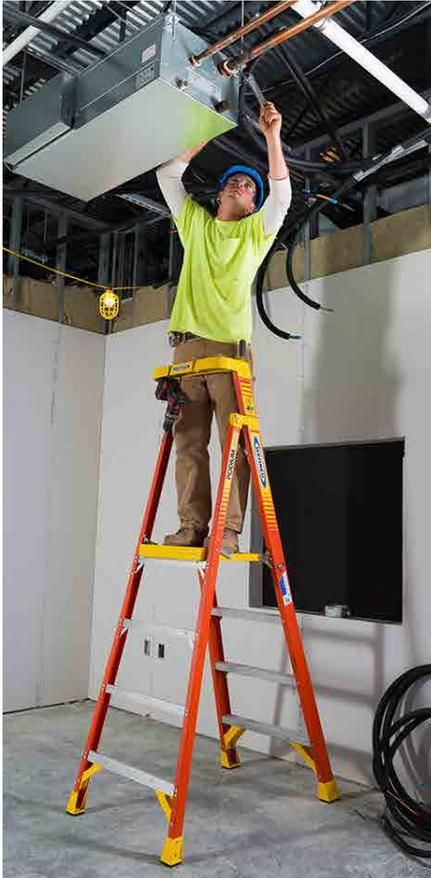
Because of the risk of electric shock, a fiberglass ladder should be used whenever working with or near electrical wires.
