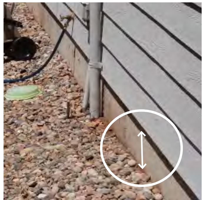
Example of good ground-to-siding clearance.
