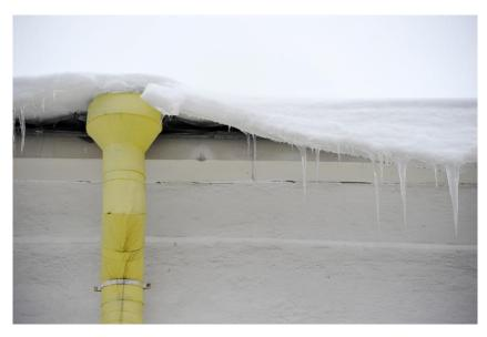
If drains are not able to operate properly, ice dams (shown above) can form and cause significant interior water damage.
