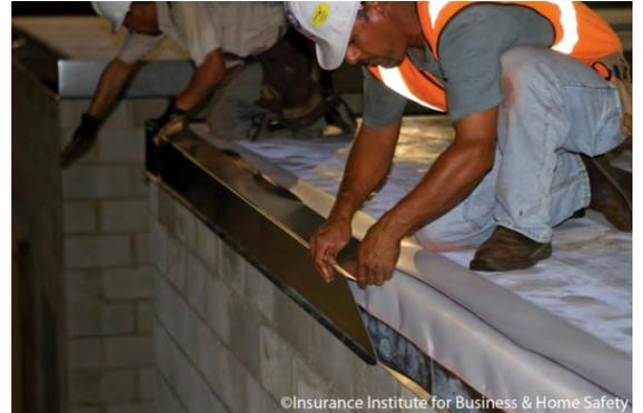
Figure 1. Metal flashing being installed over a continuous metal cleat.
