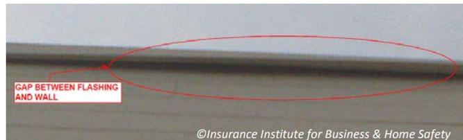
Figure 2. Roof edge flashing with gap between flashing and wall.
