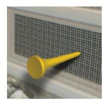
Tips: (1) Mesh can be placed on the inside or outside of the vent. (2) You can use a golf tee to test whether the mesh is the correct size of 1/8 inch or finer. If the tee does not fit through the mesh openings, it is the correct size.
