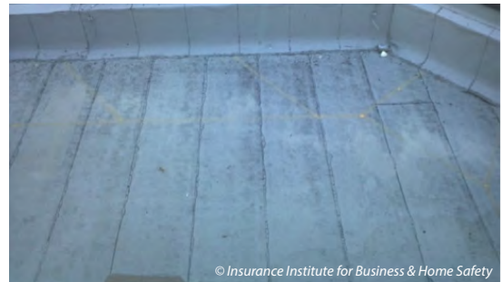
Modified bitumen roof cover.
