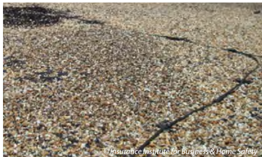
Built-up roof cover with gravel embedded in asphalt. (A lightning protection cable also is shown.)
