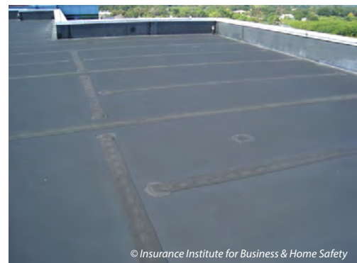
Single-ply EPDM membrane roof cover (mechanically attached).
