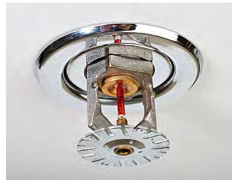
Pendent sprinkler head with glass bulb.
