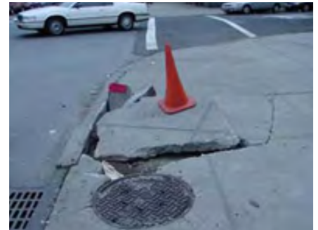
Collapsed sidewalk
