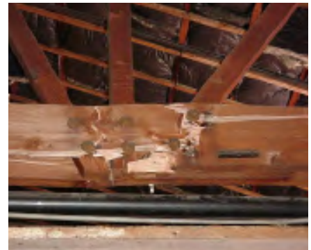
A tension failure has resulted in the bottom chords becoming fractured and pulling apart. This ultimately caused the top curve of the truss to drop significantly.
