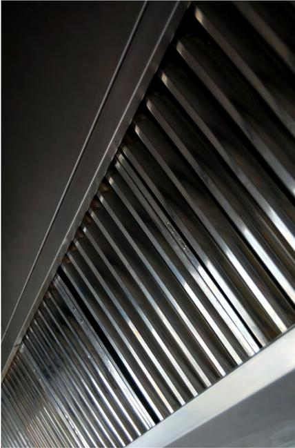
Kitchen grease filters should be tight-fitting, designed for easy removal and installed at a 45-degree angle from horizontal.
