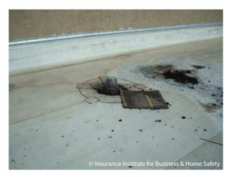
Shown is an example of an interior roof drain that is blocked by leaves and a piece of wood left behind by a contractor.
