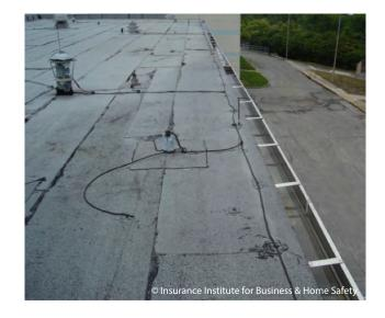
An example of a modified bitumen roof cover with aluminum gutters free of debris (including the granules from the roof cover system).
