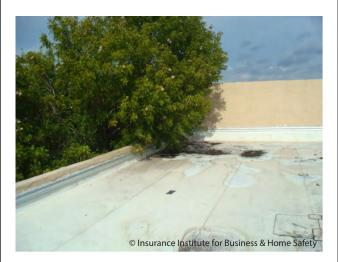
Above is an example of poor tree maintenance which can lead to leaves and twigs clogging the roof drains.
