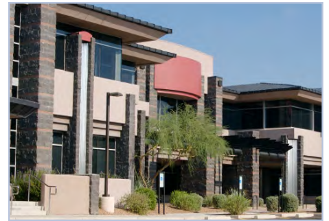
Vegetation too close to windows.
