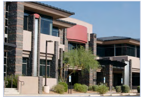
Vegetation too close to windows.
