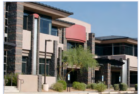
Vegetation too close to windows.
