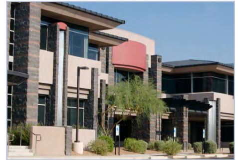
Vegetation too close to windows.
