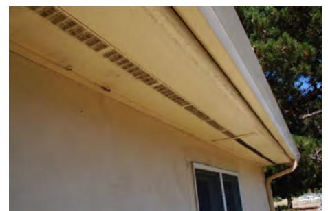
Open eave (top photo) and soffited eave (bottom photo) construction. Source: firecenter.berkeley.edu/bwmg/soffit-eave-1.html
