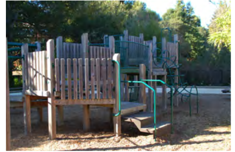
A wood play structure. Note the larger wood members in this play structure. The bark mulch used for the surfacing material pose a bigger threat in terms of ease of ignition from an ember exposure. Source: Stephen L. Quarles
