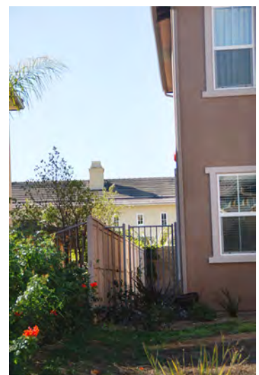
A gate made from noncombustible materials should be used where a connection is made to the house. Source: firecenter.berkeley.edu/bwmg/attachments-1.html
