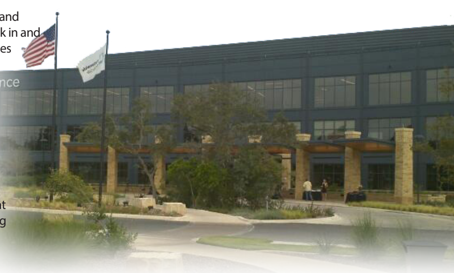
This Nationwide Insurance call center, completed in 2012 in San Antonio, Texas, was the first structure built using the FORTIFIED for Safer Business standards.
